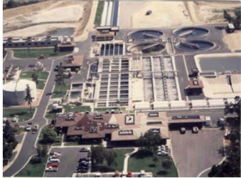
Simi Valley Water Treatment Plant
